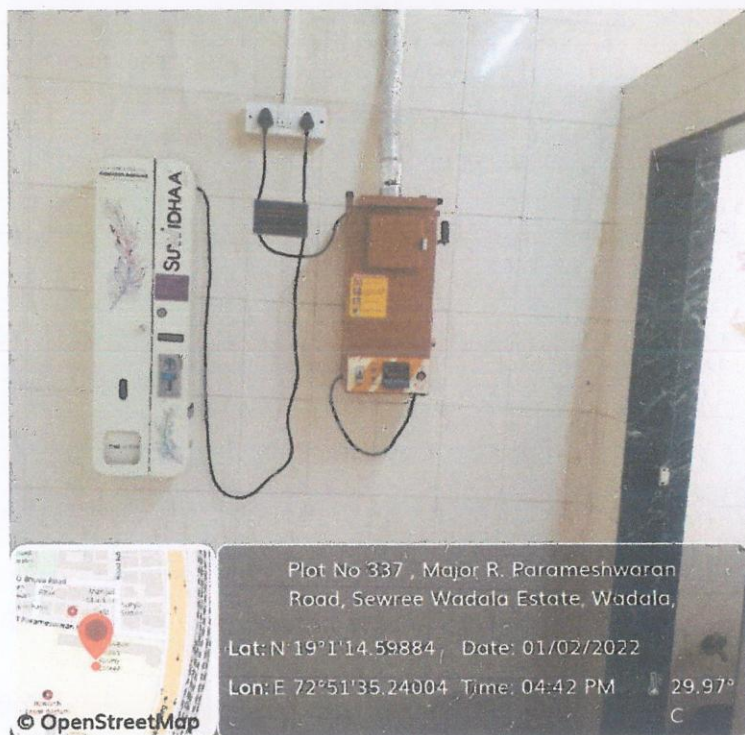
Sanitary pad vending machine and incinerator in Ladies' washroom on third floor, Central building
